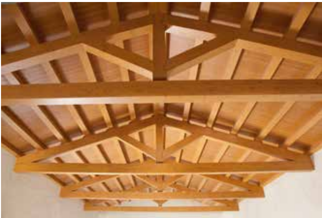
ROOFS: Traditional carpentry elements of small and medium size with highly precise joints.
