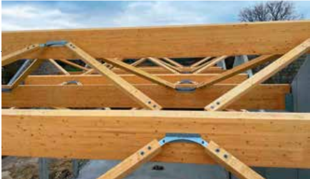
LARGE BEAMS: Structural elements in glulam of medium and big size, characterized by cuts, joints, mortises and holes to be realized with high precision.
